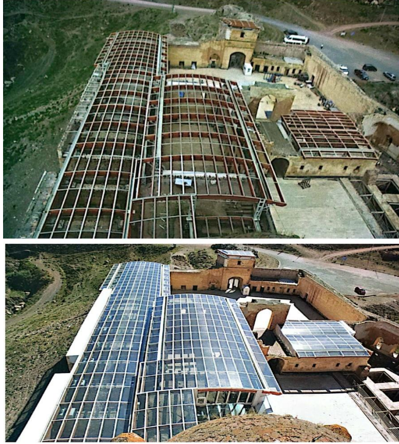
Fig.6. Glass-covered wooden roof (Belli, 2012:84)
